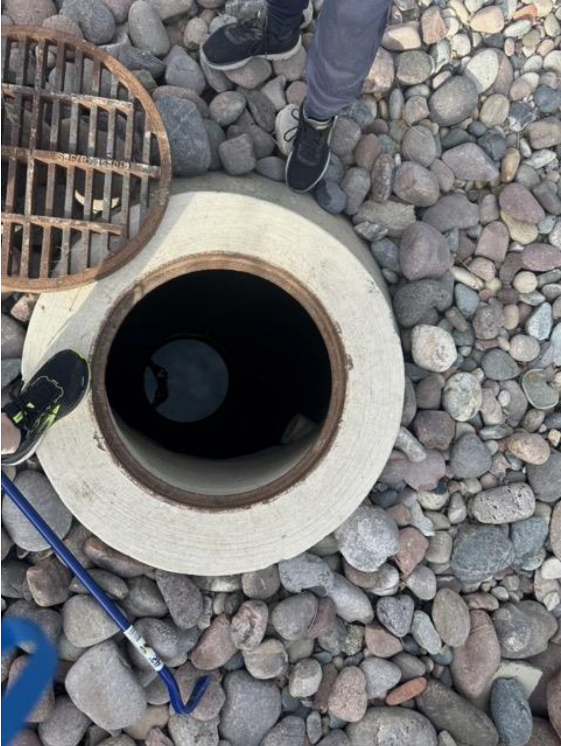
Montage Drywell Manhole
