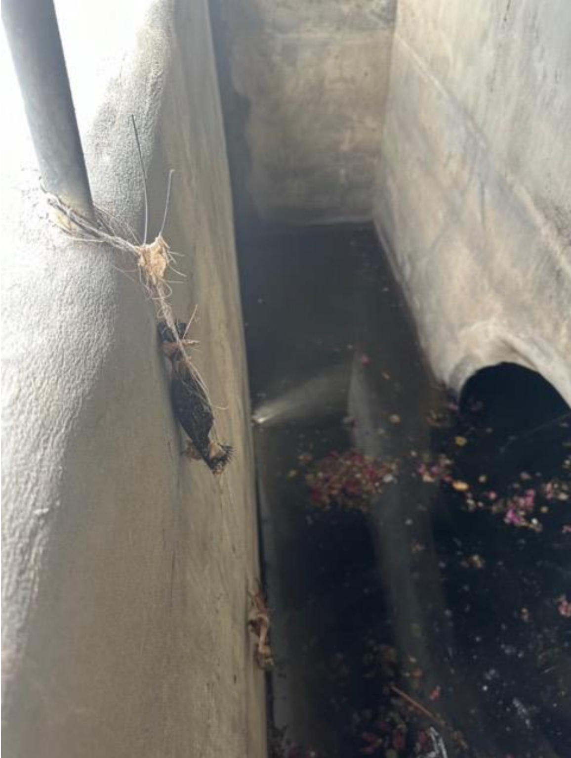
Inside East Stormwater Box Culvert and Connecting Drywell Inlet Pipe.
