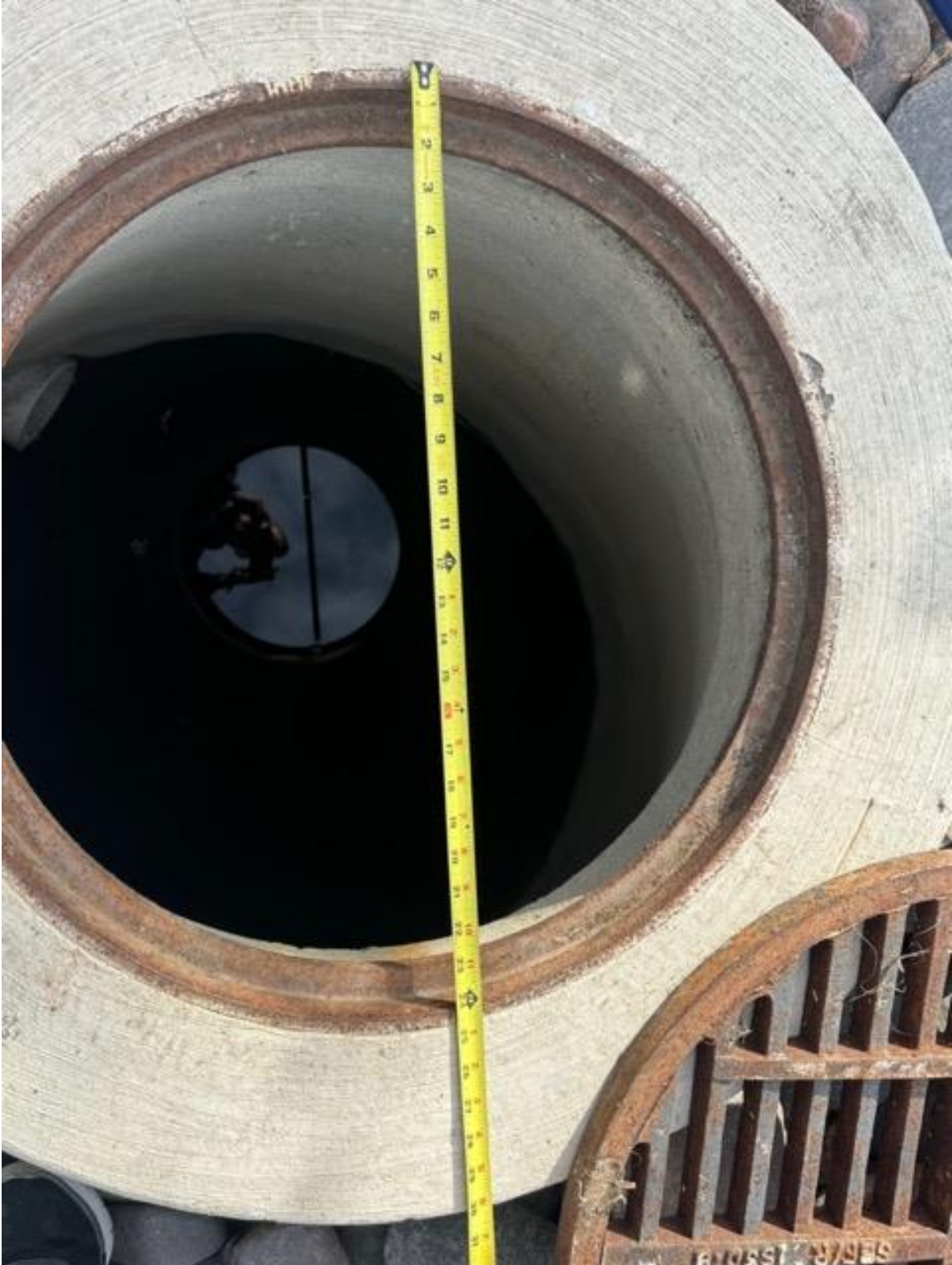
Montage Drywell Manhole
