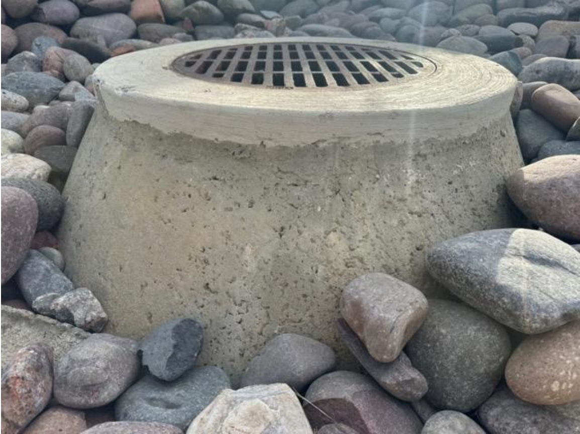
Montage Drywell Manhole
