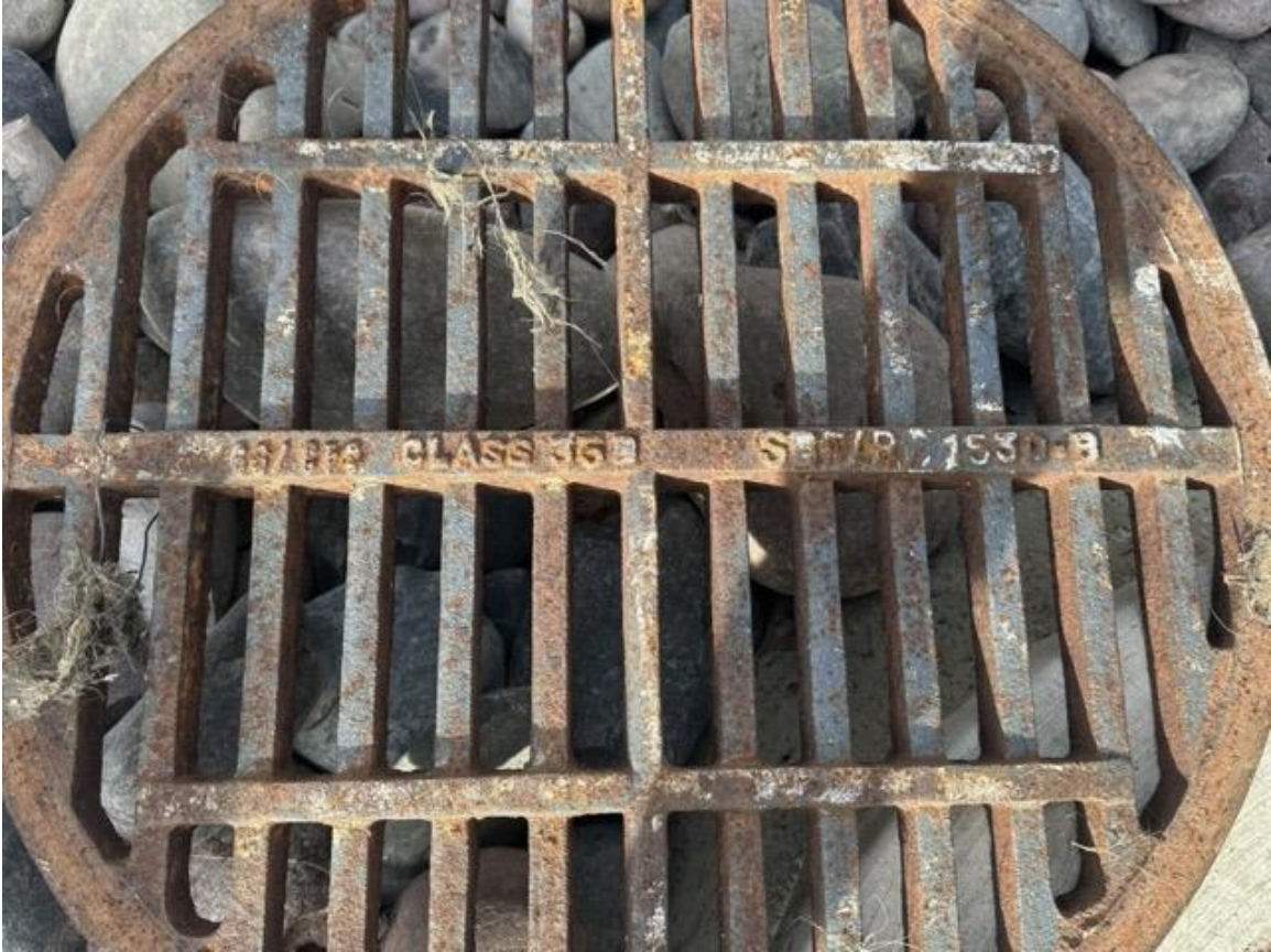
Montage Drywell Manhole
