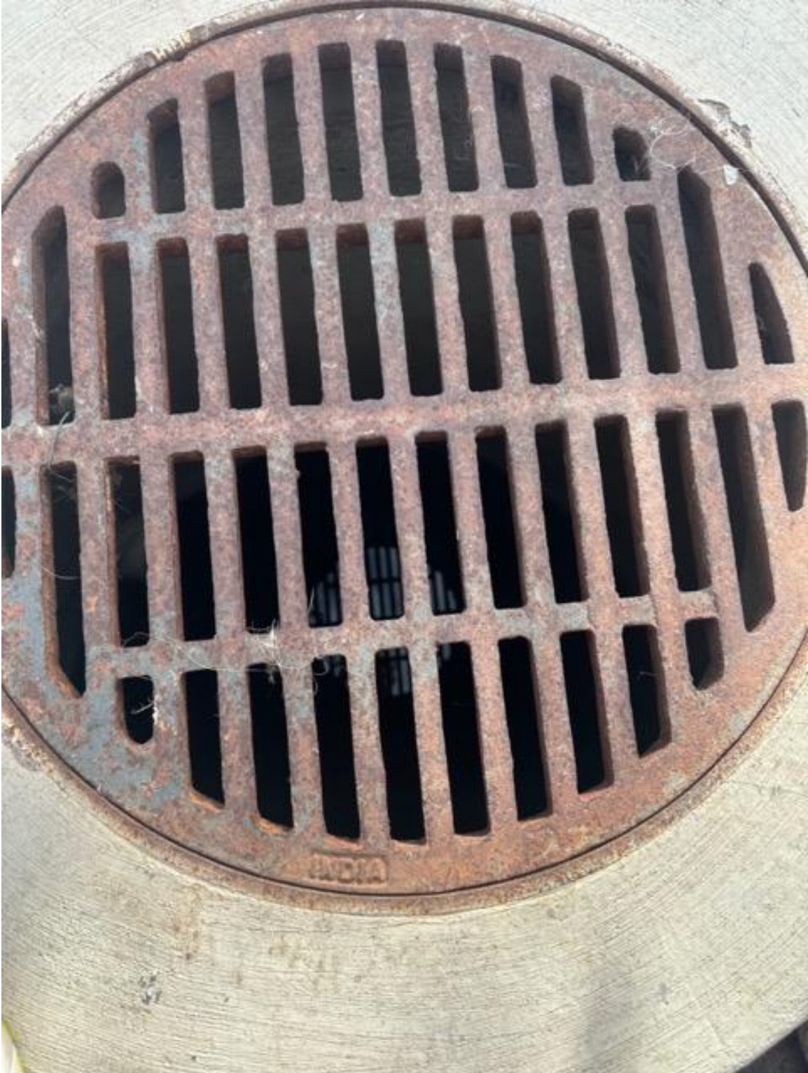
Montage Drywell Manhole
